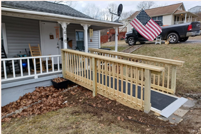
A newly-installed wheelchair ramp built through FTAAAD's Options 2.0 program.
